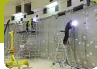
Welding in the water storage pool
