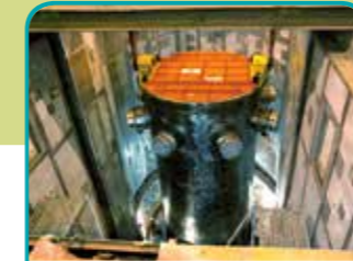
2 Reactor pressure vessel designed for a 60-year lifetime
