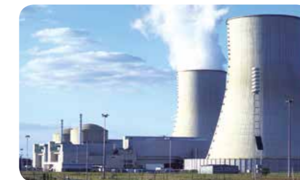
Civaux nuclear power plant, France Photo courtesy of AREVA
